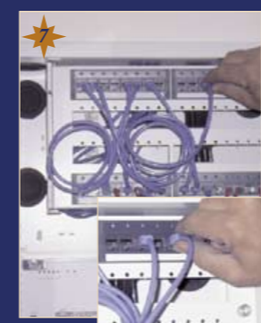
Patching in the phone and data points.
